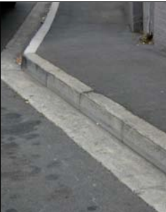
Existing concrete kerb
