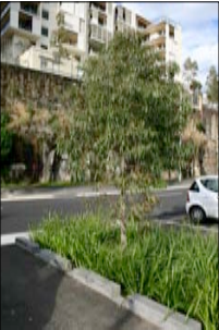
Bioswale/rain garden with tree planting
