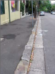
Existing stone kerb to be salvaged on site and reused on Stirling Street
