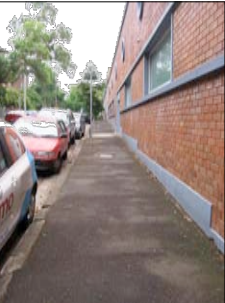
Asphalt paving on Wentworth Street
