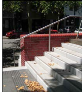
Insitu concrete steps with stainless steel railing and glazed brick retaining wall
